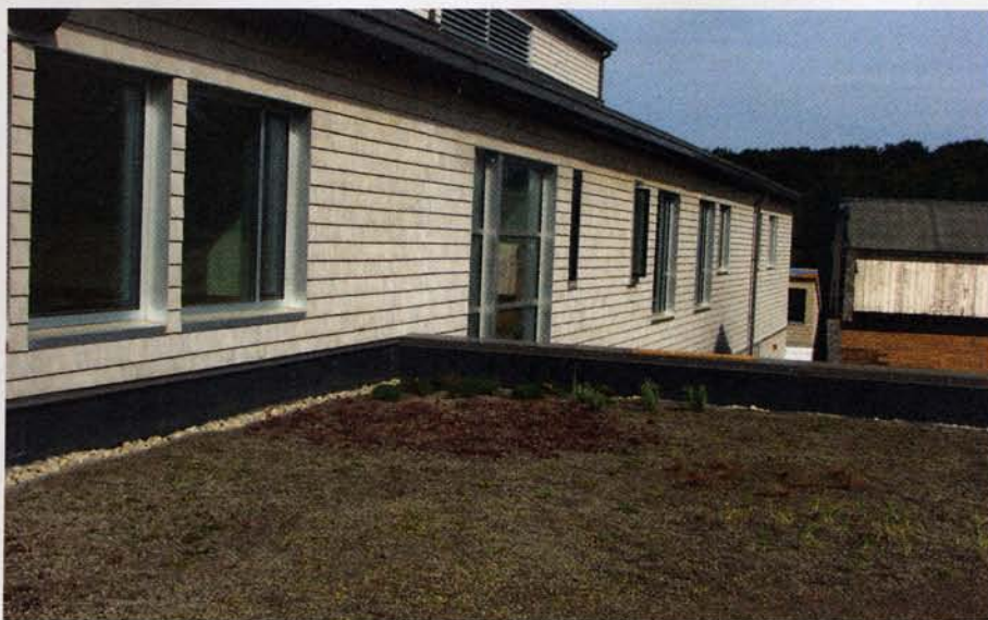
THE POTTER LEAGUE FOR ANIMALS SHELTER FEATURES A VEGETATIVE ROOF FROM THE APEX GREEN ROOF CO.
