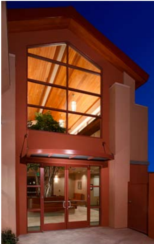
Bakersfield Veterinary Hospital (Bakersfield, CA) 13,570 SF general practice which also includes specialty, referral and emergency clinic plus luxury and general boarding.
